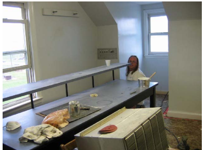
Jeff, WD8JLI doing a great job on the radio room
